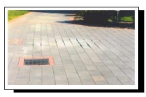
As managers we suggested a fresh approach using Koukourou Engineers and Michael Hutton from Lynch Meyer lawyers. The engineer's report revealed that the builder had failed to lay a proper foundation (to Australian Standards) for the pavers resulting in them moving and coming loose. The poor backfill and compaction had also caused the crushing of plastic storm water pipes and sumps.
