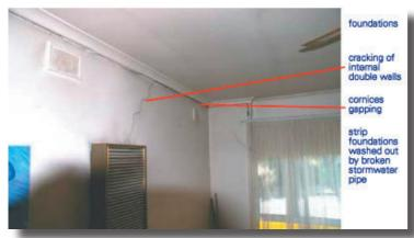
One modern group of apartments in North Adelaide found the solution to building movement and cracking caused by drying soils was to install a deep soil watering system. This uses drippers and slotted pipework below the soil surface.
