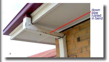
In the above photo we see rust in the downpipe serving the gutter above. This is caused by leaf and other waste laying in the pipe over years.
